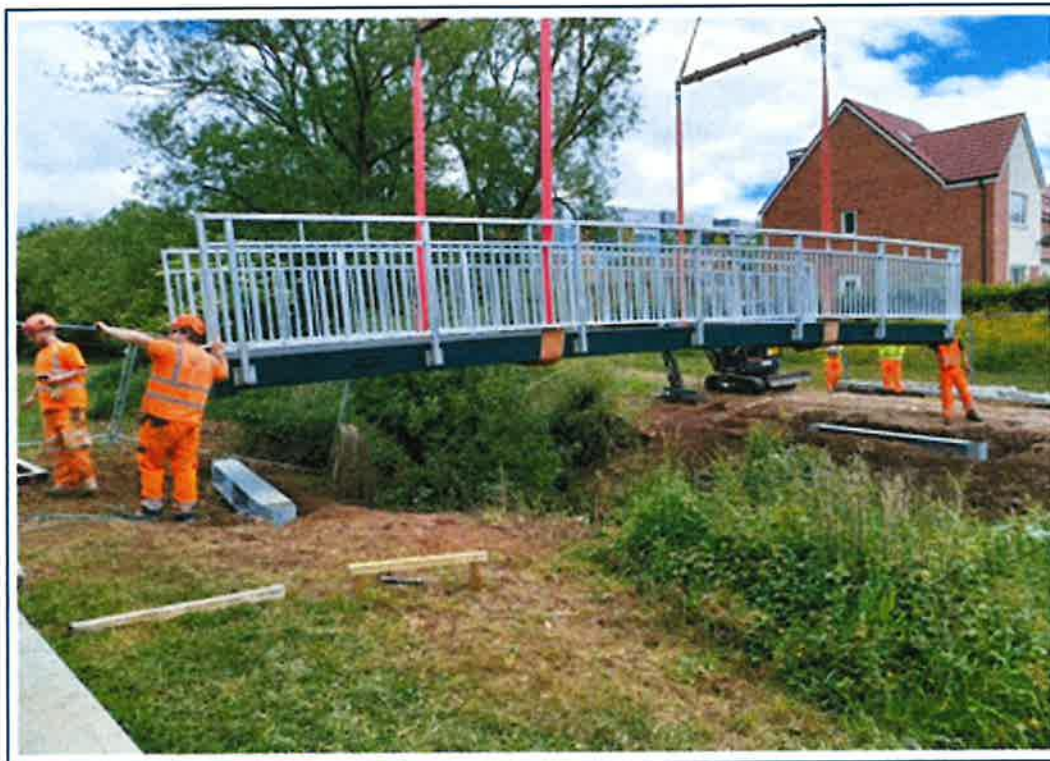
Figure 1-2 - Example Bridge Construction
